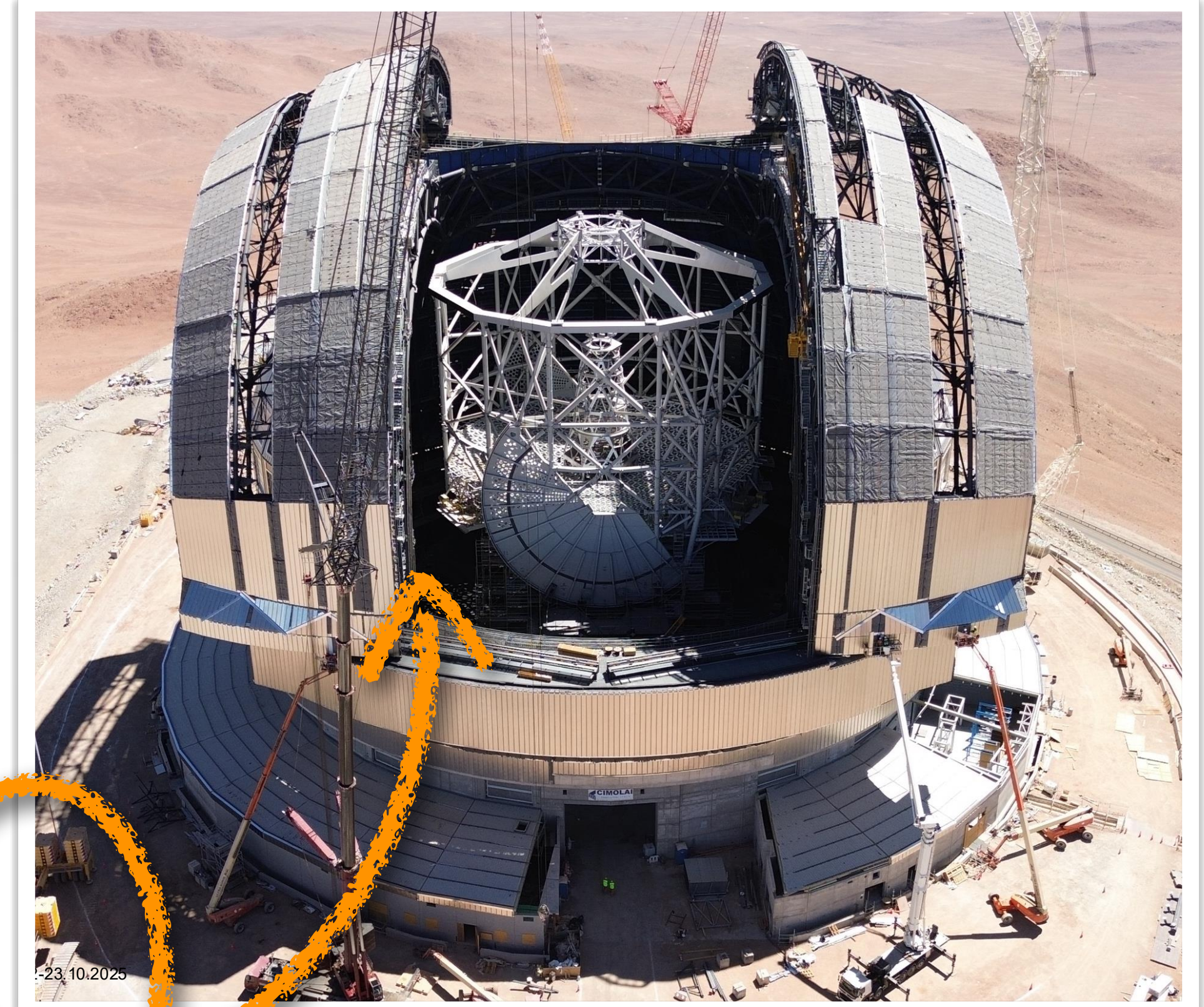
ELT construction 70% completed
